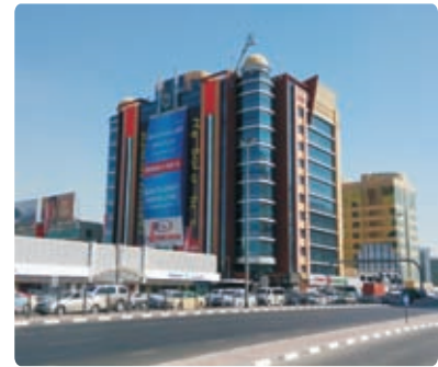
The UAE Regional Sales and Service Center
