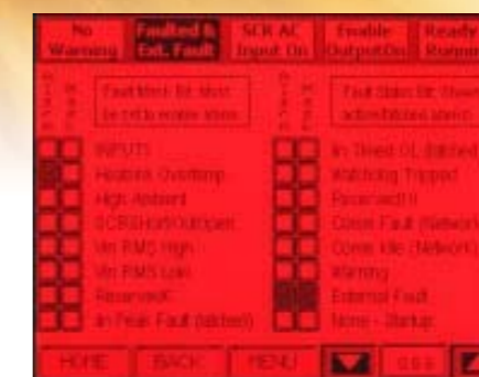
The touch screen's HMI software has user configured fault conditions.
